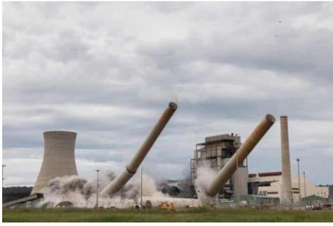
Explosive engineers have demolished two giant chimney stacks and a boiler at a defunct coal-fired power station west of Sydney as part of efforts to transform the site.
